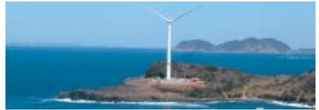
Kushizaki Wind Power Station in Chinzei Town, Higashi-matsuura-gun, Saga Pref. (1,980 kW, subsidized in FY2003)
