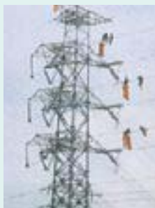
Wind noise reduction work on 220 kV transmission lines
