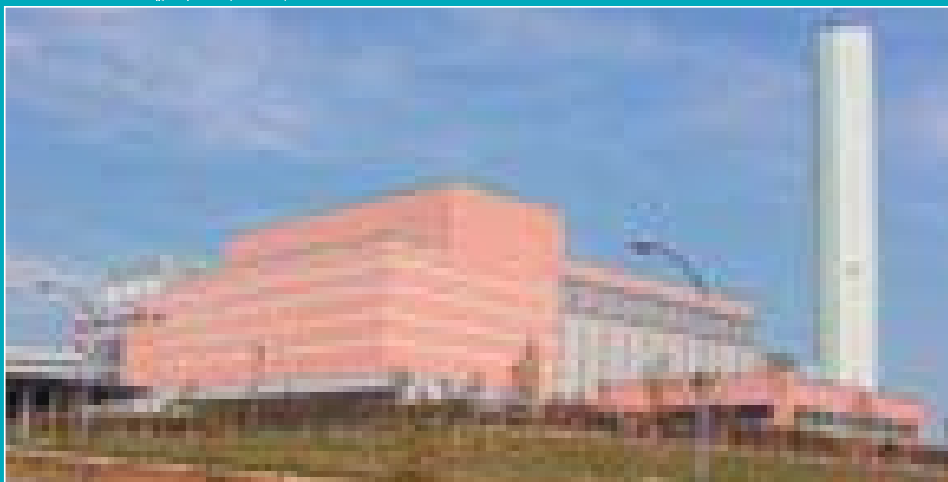
Fukuoka Clean Energy Corporation (Tobu Plant)
