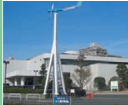
Kyushu Energy Hall
