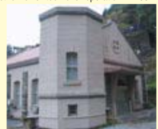
Ota Power Station
