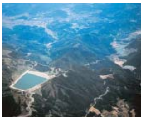
Tenzan Power Station
