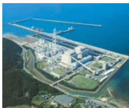
Reihoku Power Station
