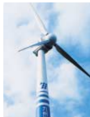
Noma wind park power station
