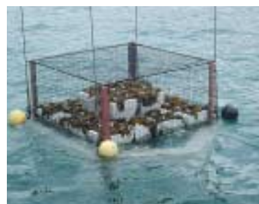
Immersion at K-hat Reef (algal reef) (Saikaiosaki, Nagasaki Prefecture) [For effective coal ash utilization, marine environment restoration]
