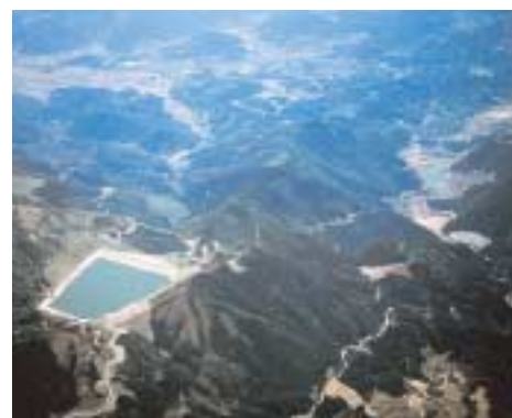
Tenzan Power Station
