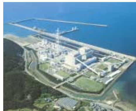
Reihoku Power Station
