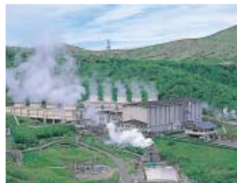
Hatchobaru Power Station
